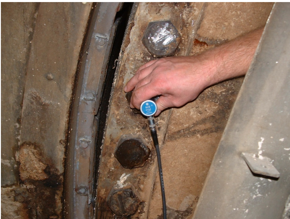
Fig. 4: bolt heads are properly cleaned for UT
